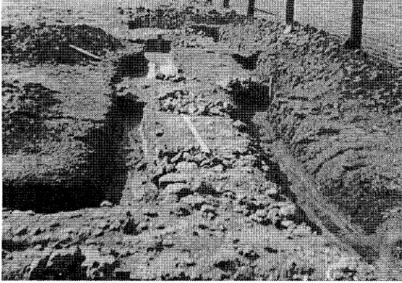
Figure 2. Stone foundations, ca. 1968. Photograph courtesy of Victoria College.
